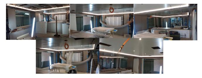
• IN GALLEY WAS INSTALLED FLOOR, START TO INSTALL ROOF CELING AND TESTED OF LIGHTS.
